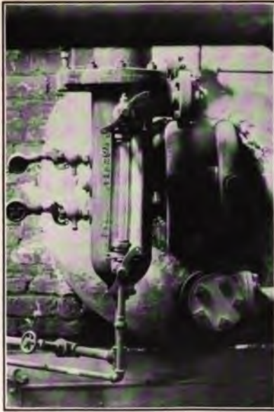
PLATES 3 AND 4.—GAUGE GLASS FOR INDICATING HEIGHT OF WATER IN A BOILER
